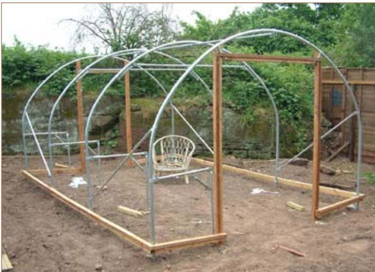
Kevin's polytunnel mid build: note the chair already installed!
